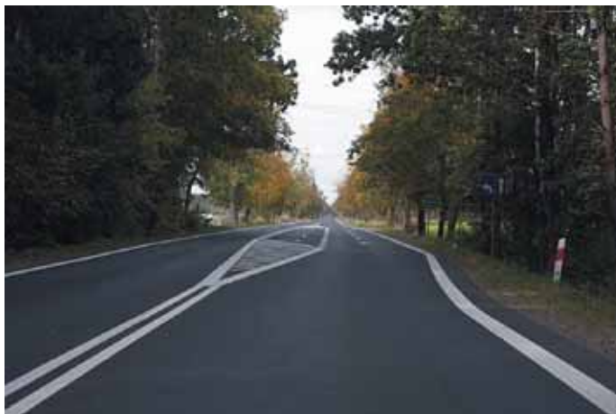
Photograph 7. On the Magnuszew – Ryczywół section, even at minor junctions, short turn-lanes were sectioned off, which prevents the blocking of traffic and reduces the number of collisions and accidents
