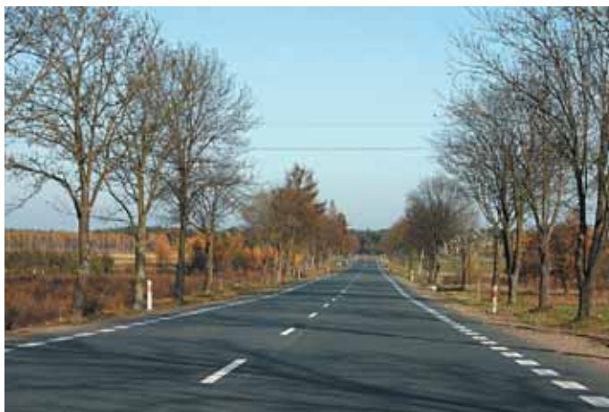
Photograph 5. The Bałtówka – Annopol section includes straights which allow overtaking.
