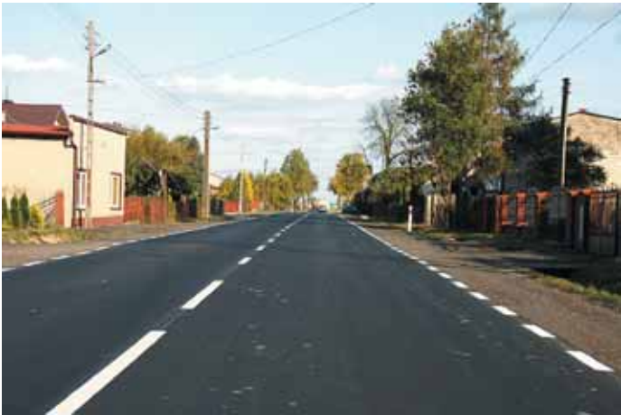
Photograph 1. The potential reference section Brzeźnica Nowa – Radomsko on DK 42 was eliminated as a result of the field visit due to the partial replacement of road surface.
