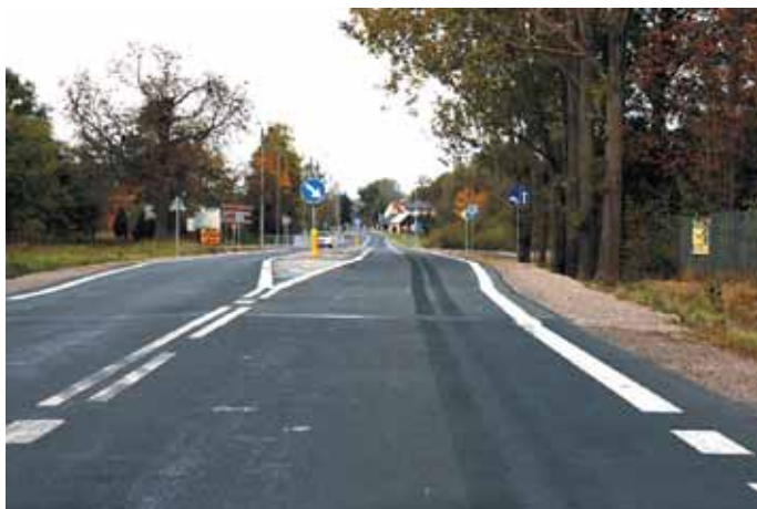
Photograph 8. Within built-up areas – especially in the Magnuszew village, being the HQ of the commune office – many islands and pedestrian refuges were placed to calm the traffic
