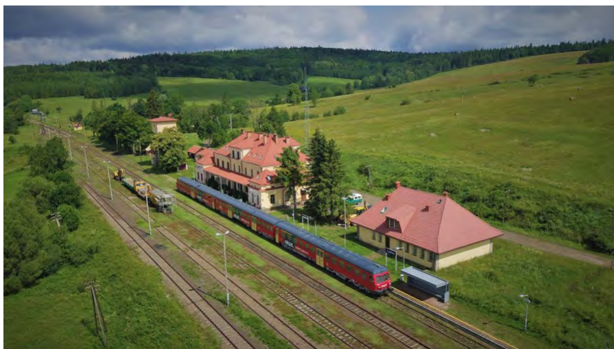
Figure 6.8 Łupków border station, Railway line 107
