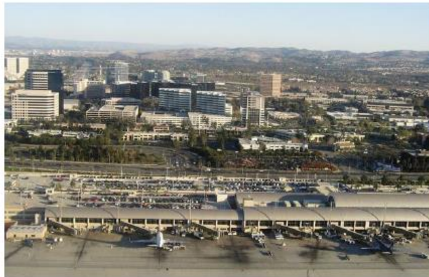
John Wayne Airport in Orange County
